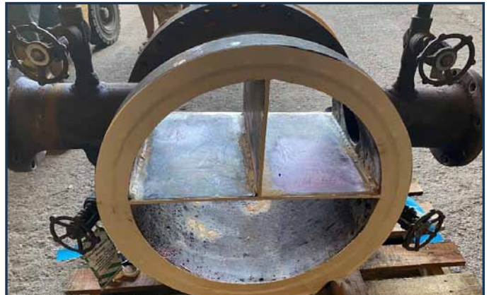
Channel, with new pass plates welded-in, masked, and ready for Curran surface prep and coating.
