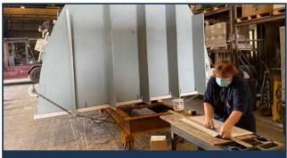
Power plant waterbox internal coating; Curran technician preparing blast mask to protect gasket sealing surfaces prior to grit blast surface prep and application of Carboline epoxy.
