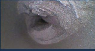
Salt water sediment and deposits severely fouled many of the condenser tubes requiring hydro lancing to clear.
