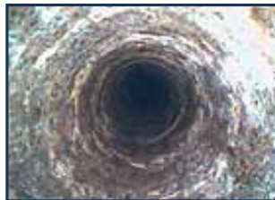
Tubes after scraper cleaning
